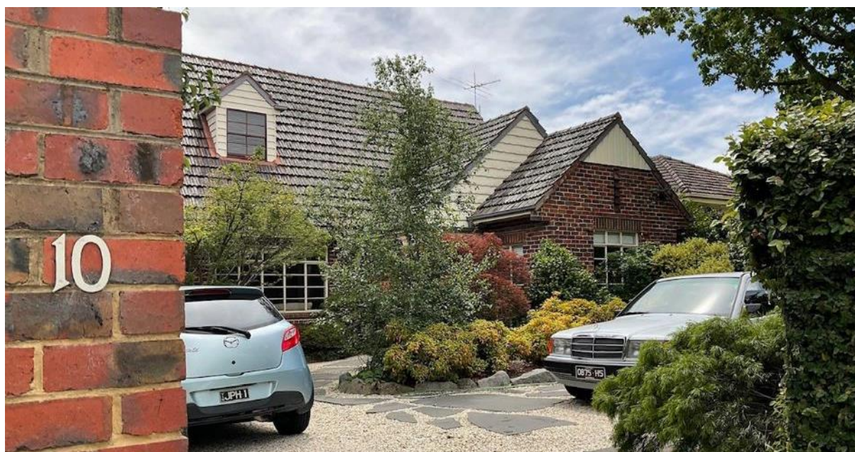
Figure 5 10 Munro Avenue, Ashburton
