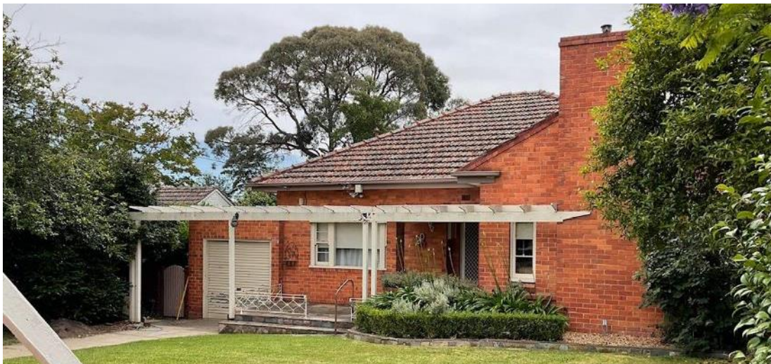
Figure 8 20 Munro Avenue, Ashburton
