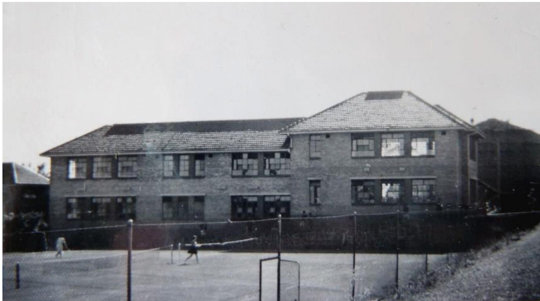
Figure 34. East elevation of the Science Block, 1955. (Source: MLC Archives).
