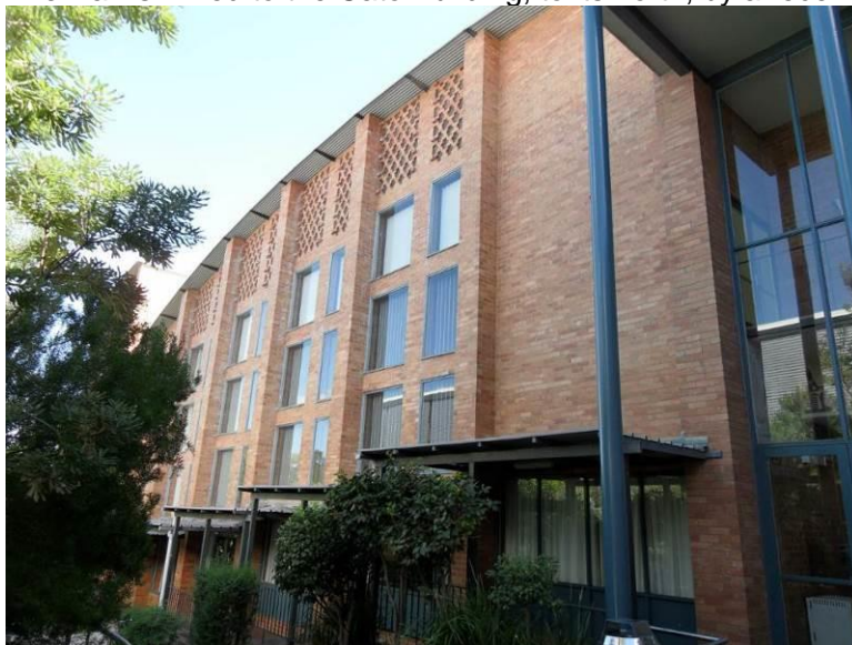
Figure 36. Nurses' Memorial Assembly Hall, east elevation. (Context, 2016)
