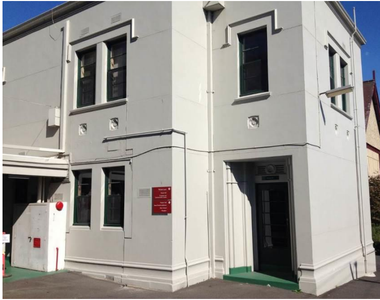
Figure 28. West end of the Boarding House Extension, looking south, 2016.
