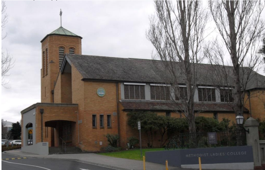
Figure 37. Fitchett Chapel, looking north-east. (Context, 2016)
