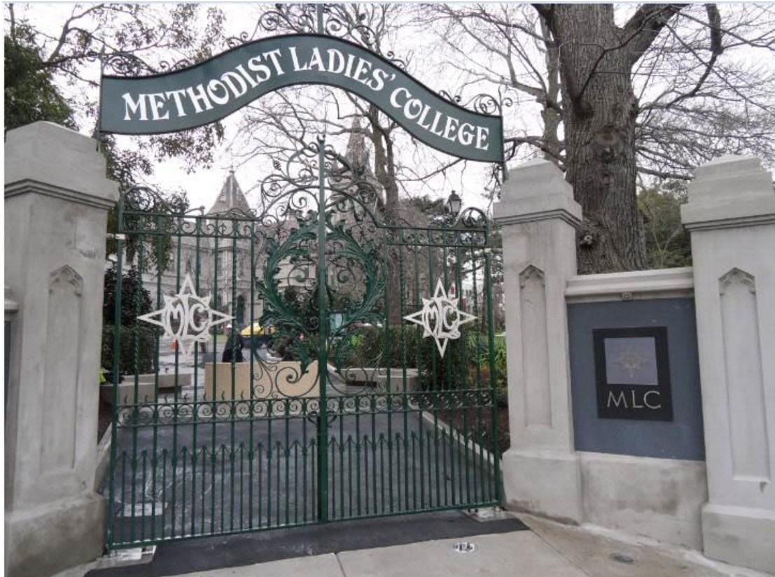
Figure 26. The Krome Memorial Gates and part of the masonry fence, 2016.
