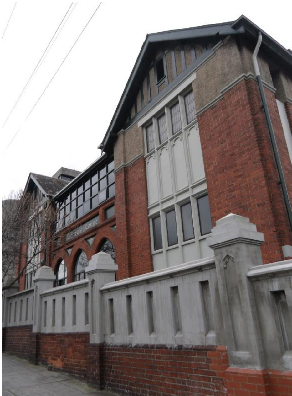
Figure 27. Nicholas House, looking north-east, 2016.
