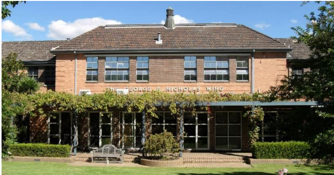
Figure 30. The east-west section of the George R Nicholas Wing (Principal's Admin area), as shown in what appears to be original metal lettering on its north elevation. Note the small cupola on the ridge. The ground floor is obscured by a later addition, but it is reportedly intact behind. (Context, 2016)
