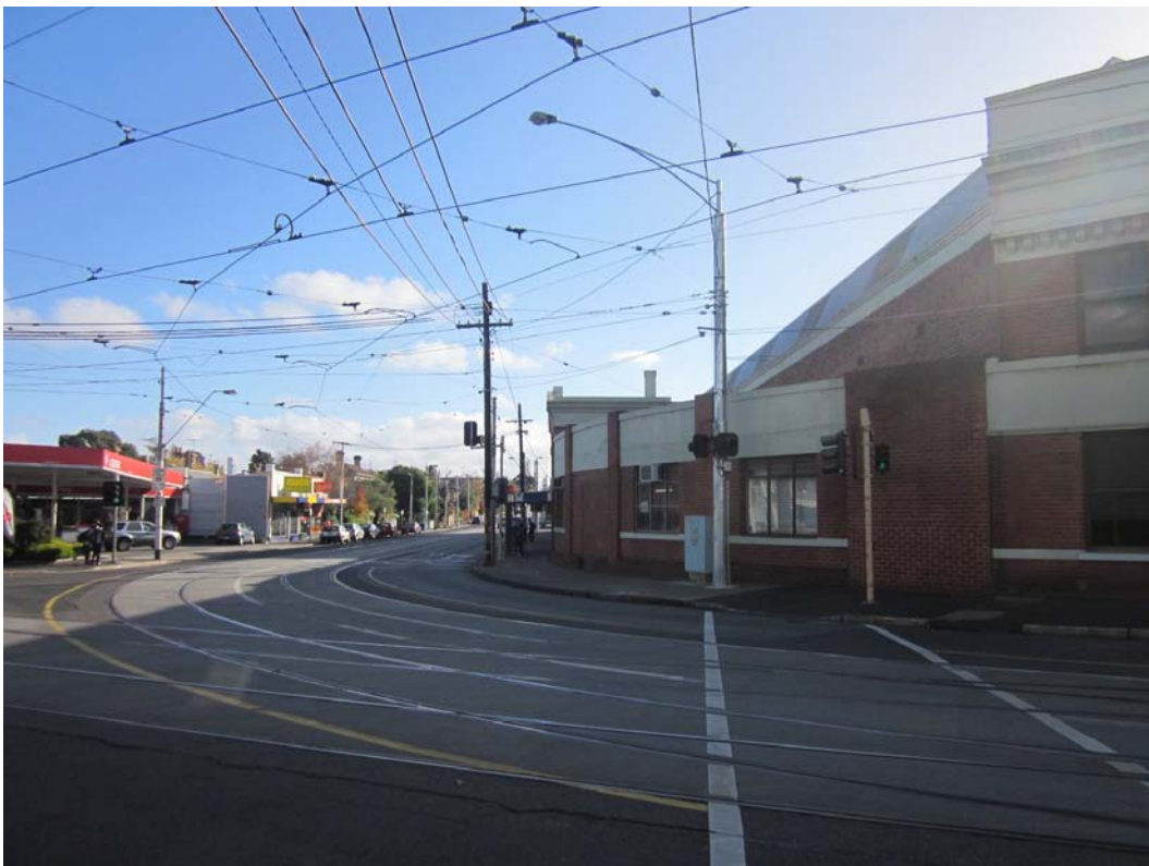
Figure 3 Single-storey infill wing at the corner of Barkers Road and High Street.
