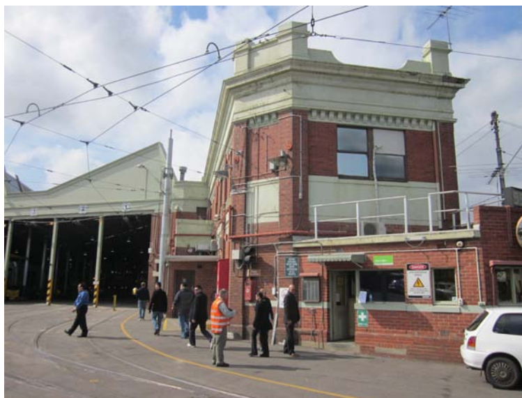
West elevation, administration building
