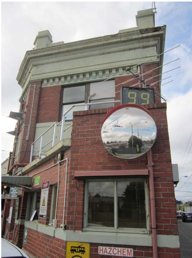
Figure 5 The Inspector's cabin adjoining the west end of the administration block to Barkers Road.
