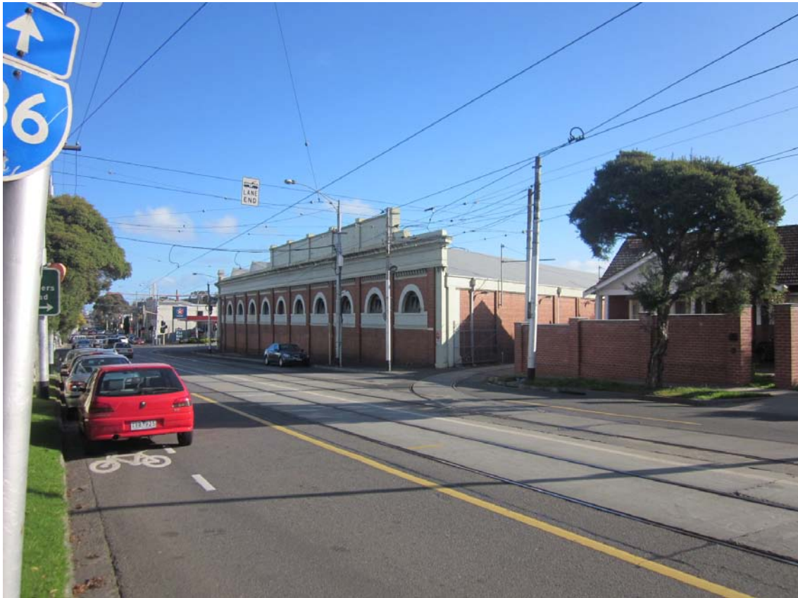
Figure 4 East and north elevations of the tram shed, view from the north-east on High Street.
