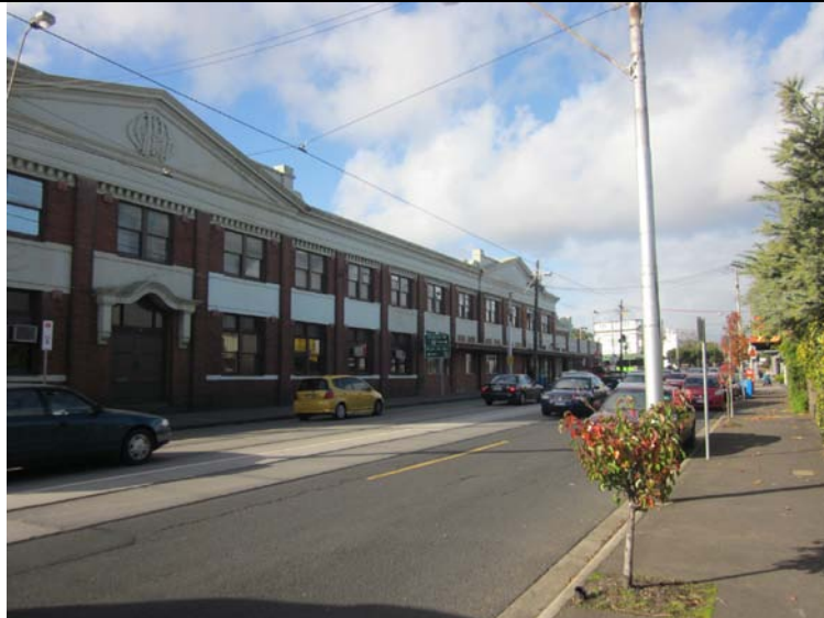
Barkers Road elevation, administration building
