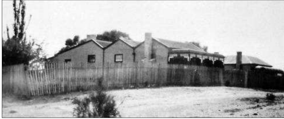
Figure 24 - The former home of Richard Pope (Mine Manager) located at 18 Daniel Street, Long Gully (just outside the study area) was burnt in the 2009 fires. (Courtesy of James Whitehead) George Ellis
