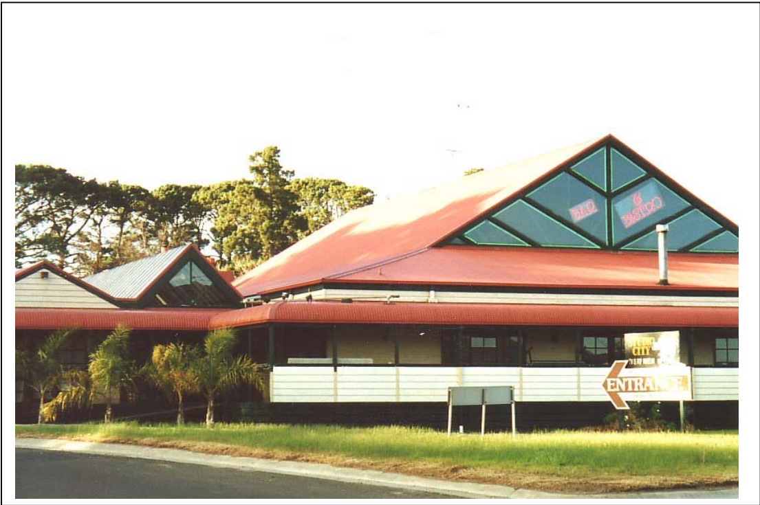
Figure 2.4.1. – Photograph showing the Coolstores frontage in 2002
