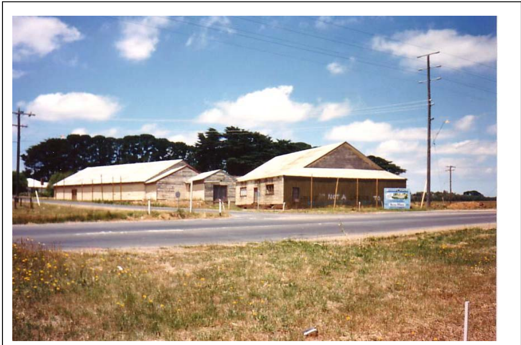
Figure 2.2.1 – Photograph showing the Coolstores and packing sheds prior to redevelopment
