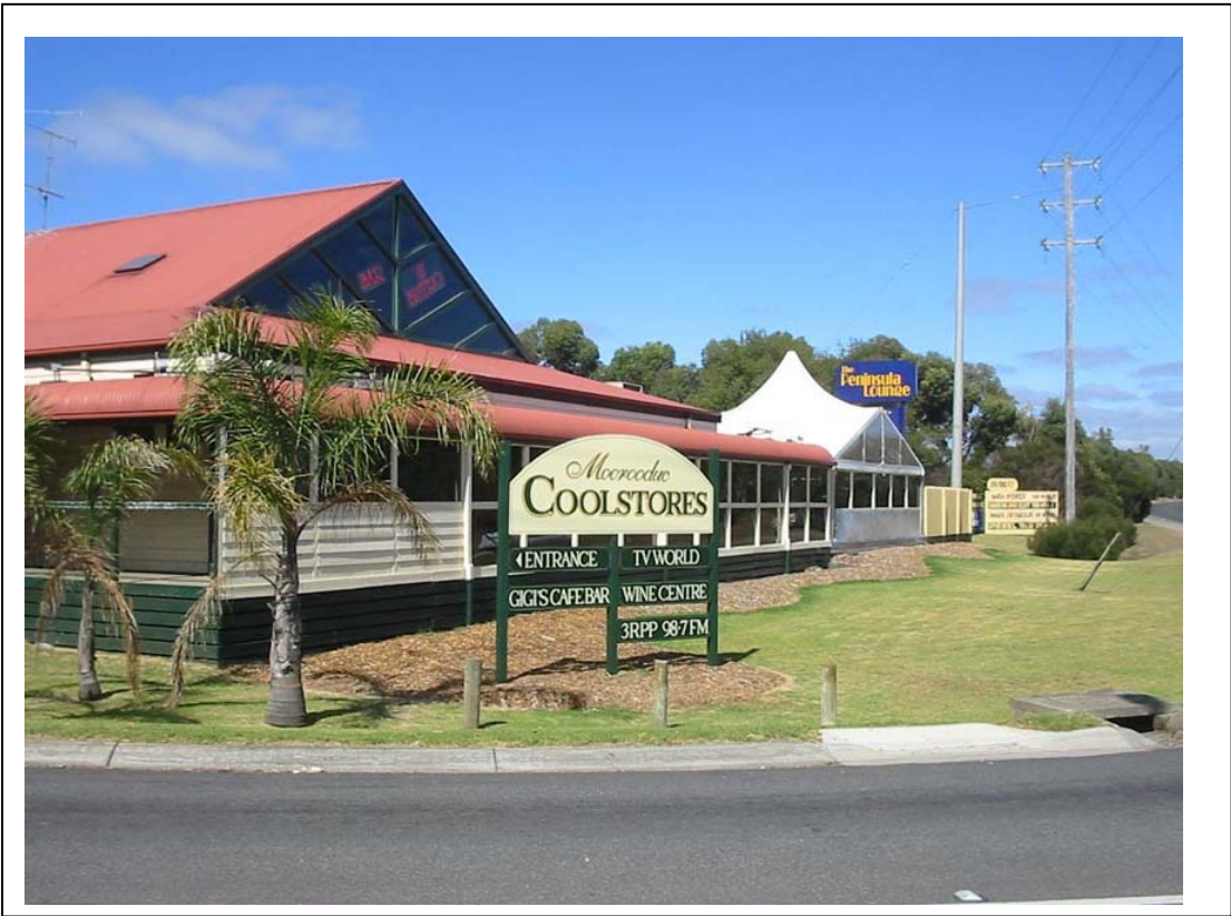
Figure 2.4.2. – Photograph showing the current Coolstores frontage
