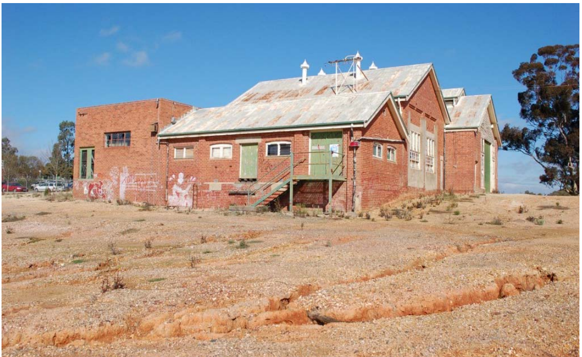
Figure 23 A similar view showing that there has been minimal changes to the brick elements. The asbestos cement sheet section has been demolished. Source: Anthemion Consultancies, August, 2011.
