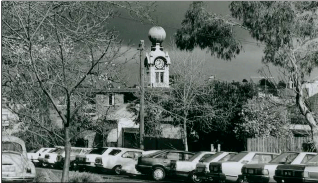
Figure 31: Dimmeys Tower, c1980s (SLV Image H2009.52/59 ).
