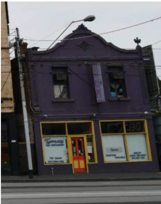
Figure 11. 30-32 Swan Street (GJM Heritage, October 2016)
