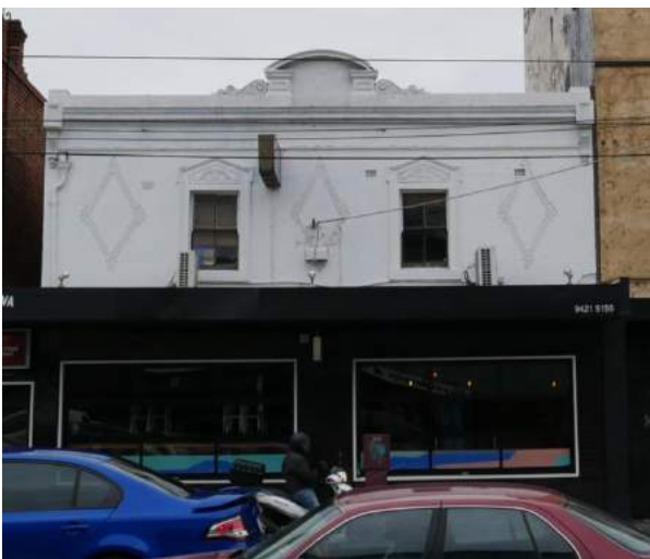
Figure 13. 36-38 Swan Street (GJM Heritage, October 2016)
