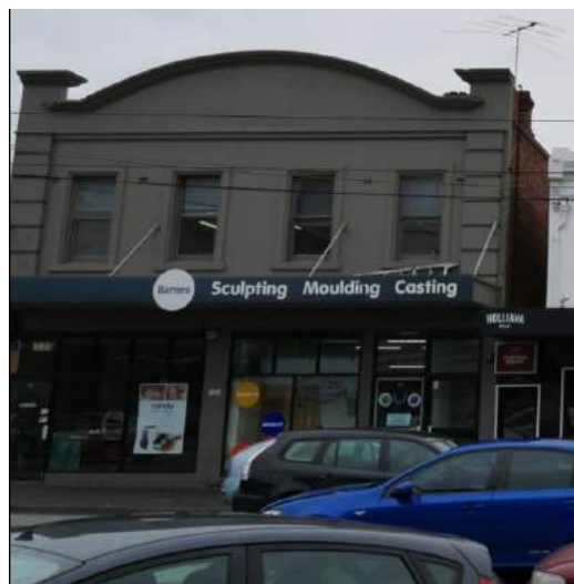
Figure 14. 40-42 Swan Street (GJM Heritage, October 2016)
