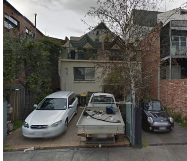
Figure 32: Rear 416-418 Church Street (Google Streetview)
