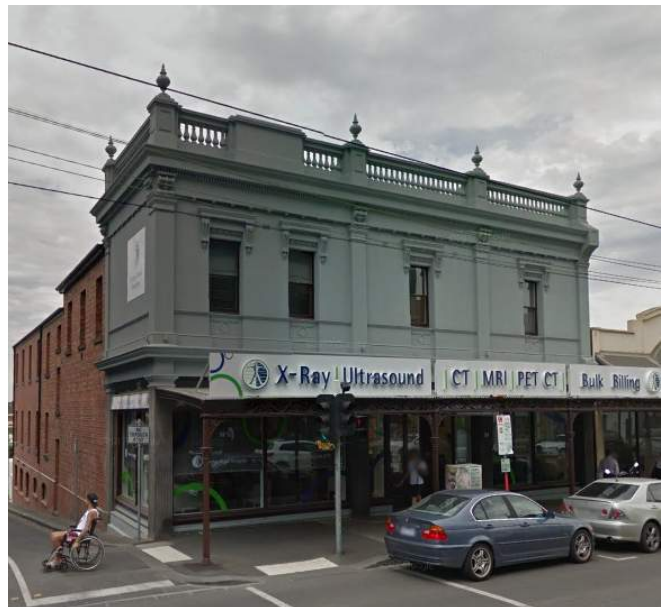
Figure 4. 84-86 Bridge Road (c1870-90), individually significant in HO310, Bridge Road Precinct (Google, Nov 2016).
