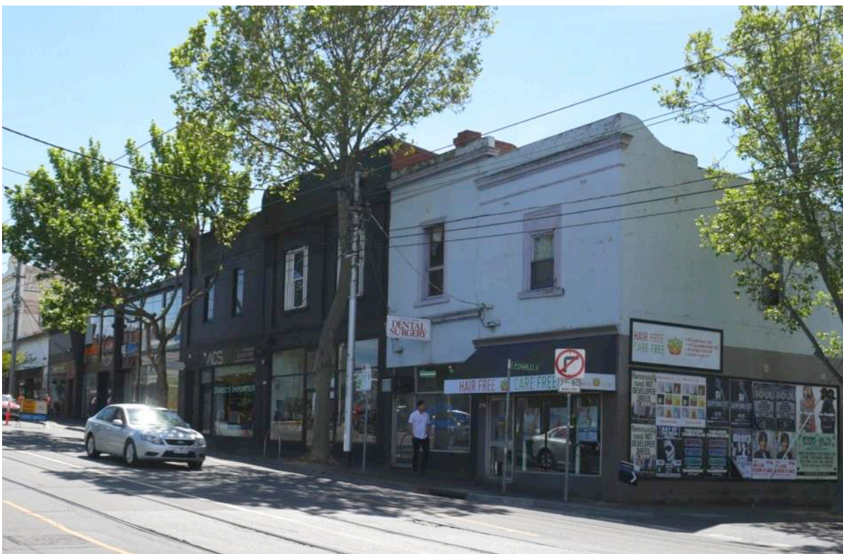
Figure 2. 223 Swan Street (L) to 235 Swan Street (R)
