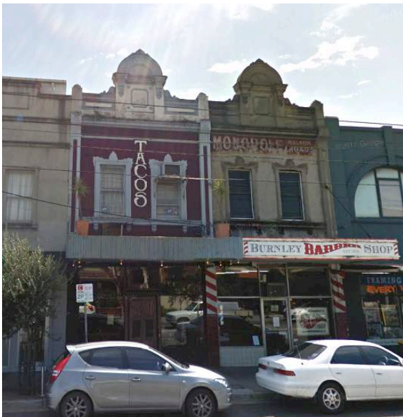
Figure 3. 413-15 Swan Street (1892), individually significant in HO474, Burnley Street Precinct (Google, Feb 2017).
