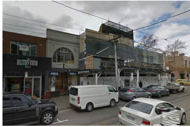
Figure 22. 127-133 Swan Street – June 2014 (Google streetview)
