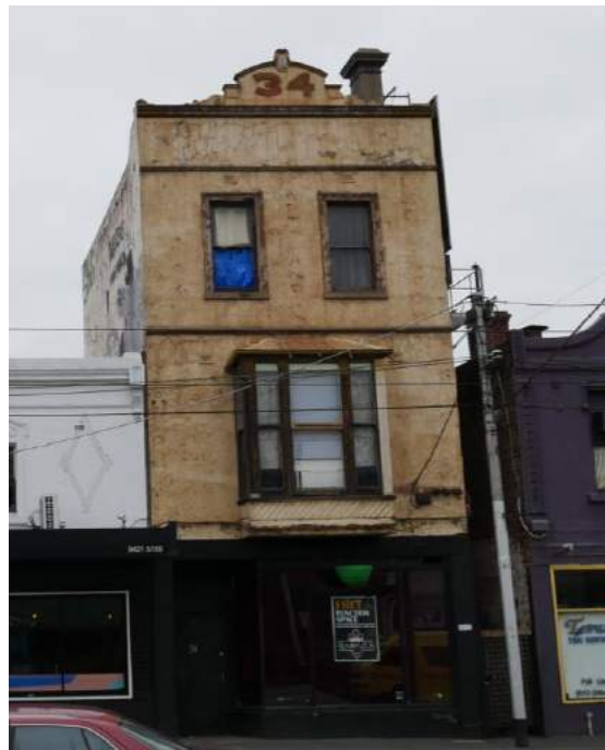
Figure 12. 34 Swan Street (GJM Heritage, October 2016)
