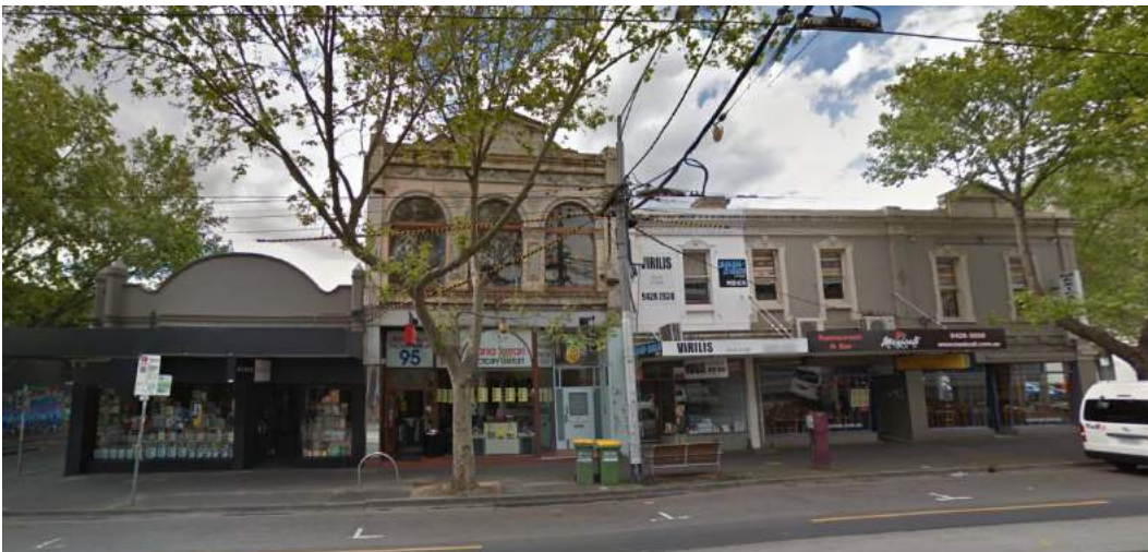
Figure 16. 91-101 Swan Street (Swan Street Precinct, HO335) (Google, Oct 2016).
