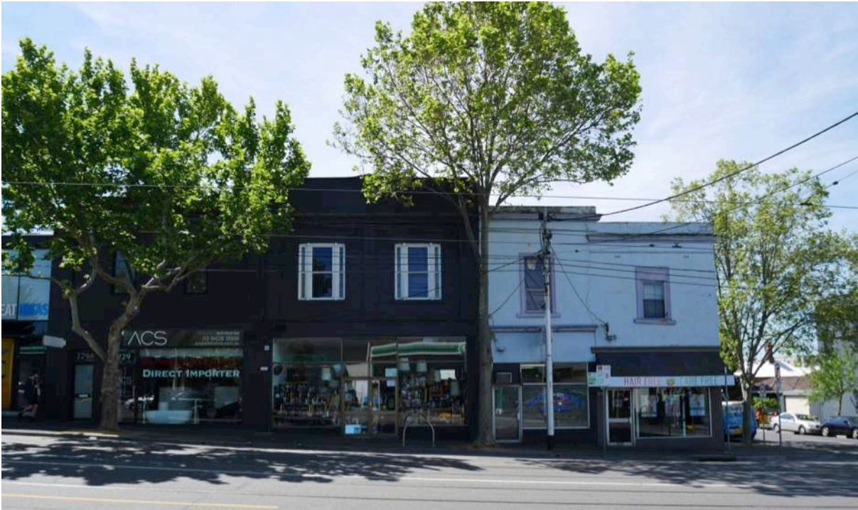
Figure 3. 229 Swan Street (L) to 235 Swan Street (R)
