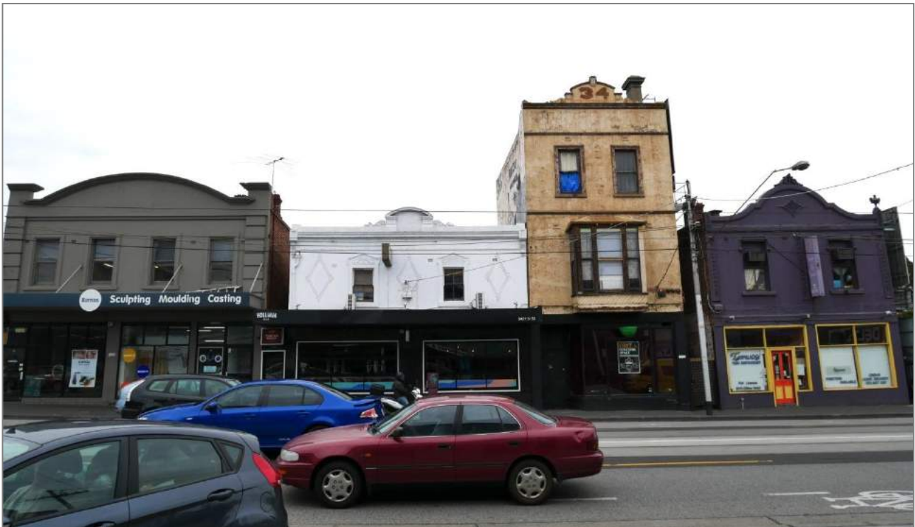
Figure 1. 30-42 Swan Street, Cremorne (GJM Heritage, October 2016)
