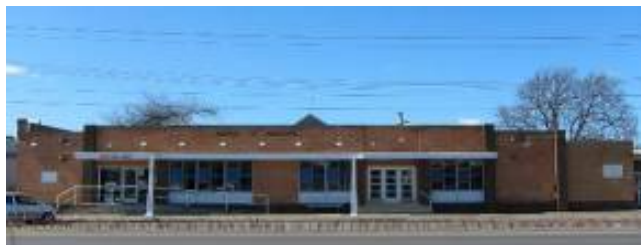
Figure 11: Former Sebastopol town hall. Source: Context 2011.
