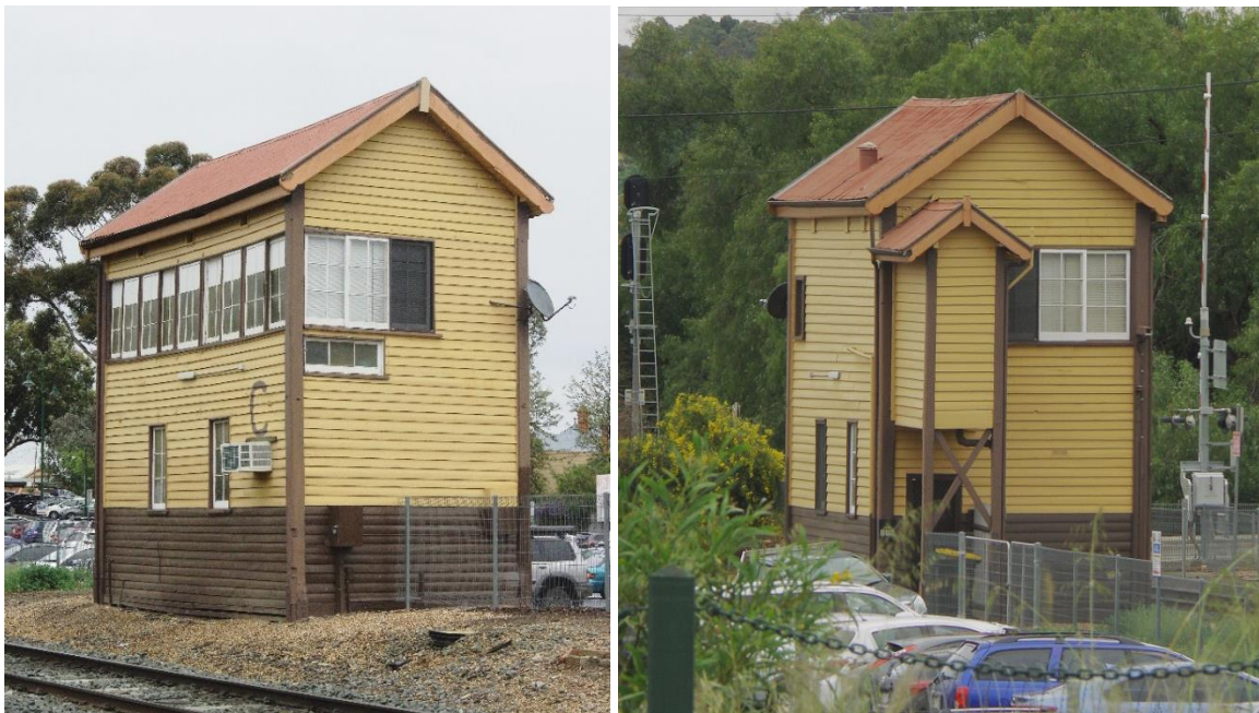
Figure 2. Former Sandhurst C Railway Signal Box viewed from southeast (left) and from northwest (right). (Source: Context, October 2019)
