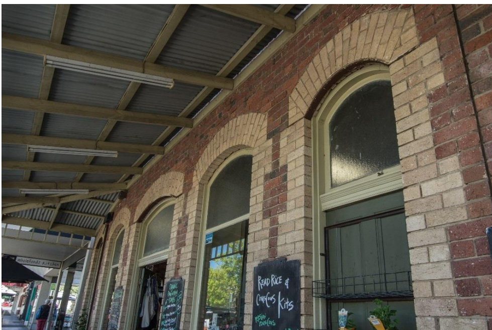
Figure 2. Ground level openings at 314 Lyttleton Terrace, Bendigo. (Source: Context, October 2019)
