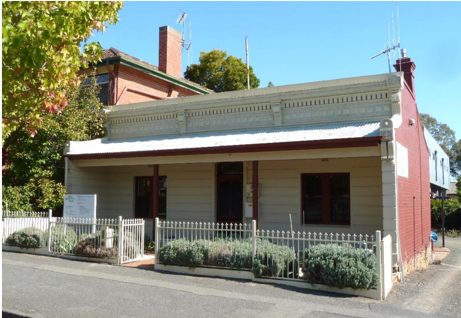
Figure 1. 56 Mundy Street, Bendigo, originally built in the 1860s as part of a row of terraced cottages and remodelled in 1880 by William C. Vahland. (Source: Context, October 2019)
