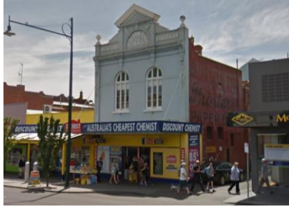
Figure 10. Former Bolton Brothers printery and stationery store, 43–45 Mitchell Street, Bendigo. (Source: Google, February 2015)
