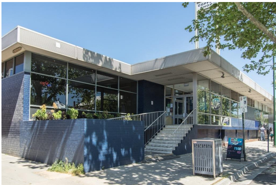
Figure 2. 159 Hargreaves Street, Bendigo, designed by architects Moore and Hammond. (Source: Context, October 2019)
