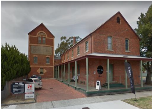
Figure 6. former Grimsby Roller Flour Mill, 35 Wills Street, Bendigo. (Source: Google, February 2015)
