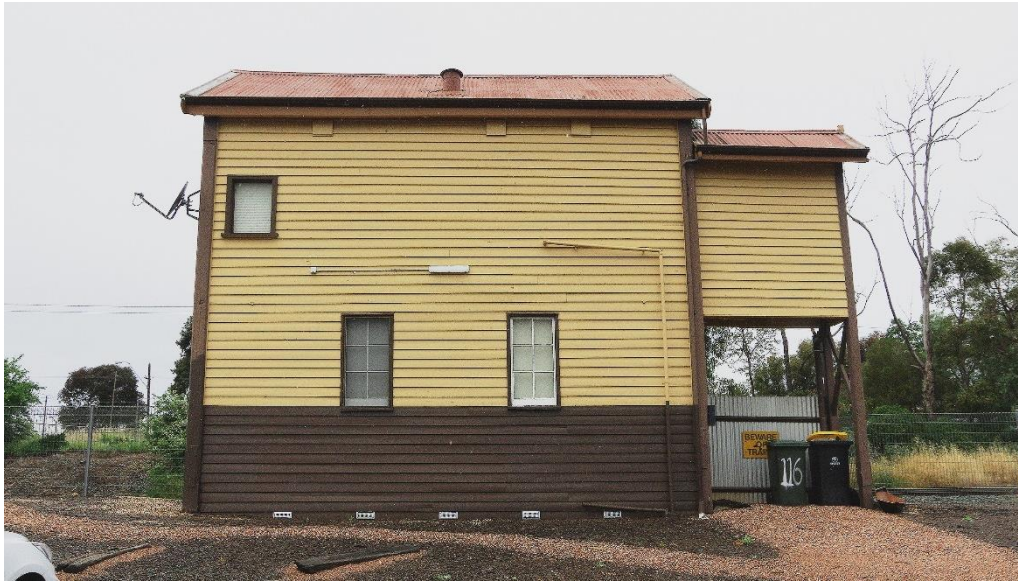
Figure 1. Former Sandhurst C Railway Signal Box at 116 Williamson Street, Bendigo, viewed from north. (Source: Context, October 2019)
