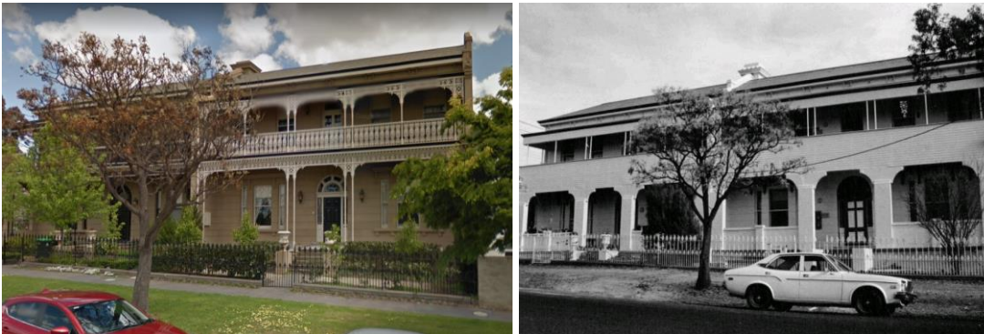
Figure 11. 121–125 Wattle Street, Bendigo, in 2016 (left) and c. 1993 (right). (Source: Google, October 2016; HERMES record no. 34426)
