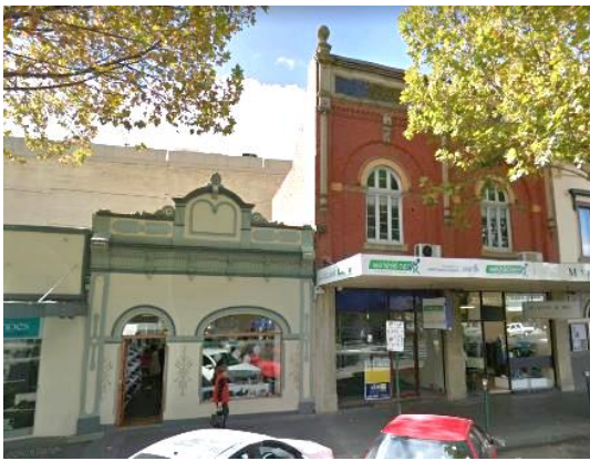
Figure 6. 33, 35 & 37 Williamson Street, Bendigo. (Source: Google, July 2017)
