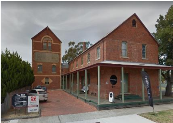
Figure 10. former Grimsby Roller Flour Mill, 35 Wills Street, Bendigo. (Source: Google, February 2015)
