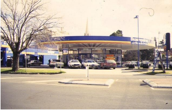
Figure 4. Former Beaurepaire Motor Garage, 404-406 Hargreaves Street, Bendigo. (Source: VHR Place ID 5380)
