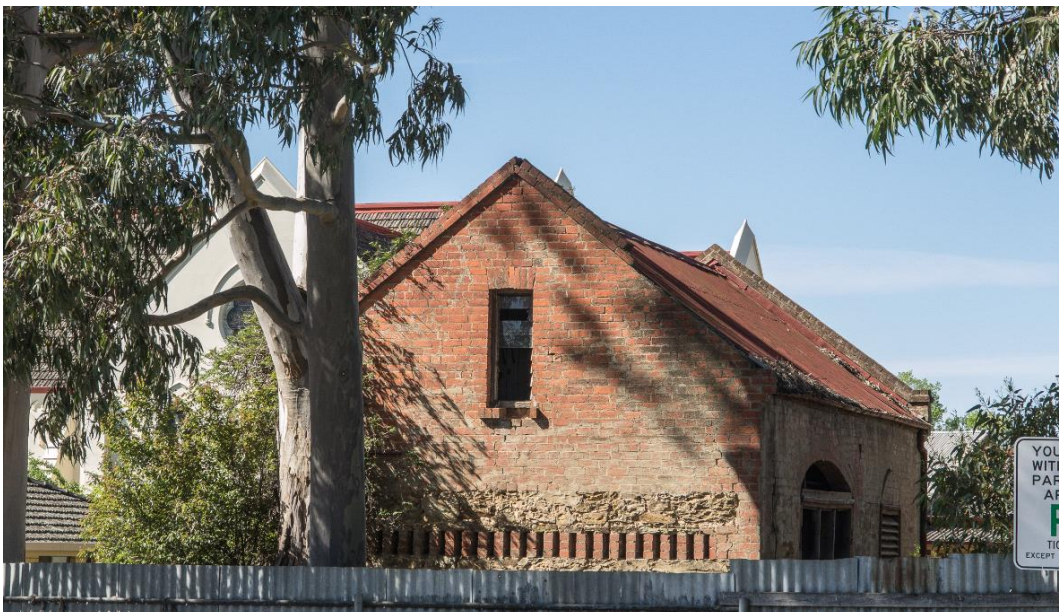
Figure 2. Southeast elevation of the stable building at 96 Mollison Street, Bendigo. (Source: Context, October 2019)
