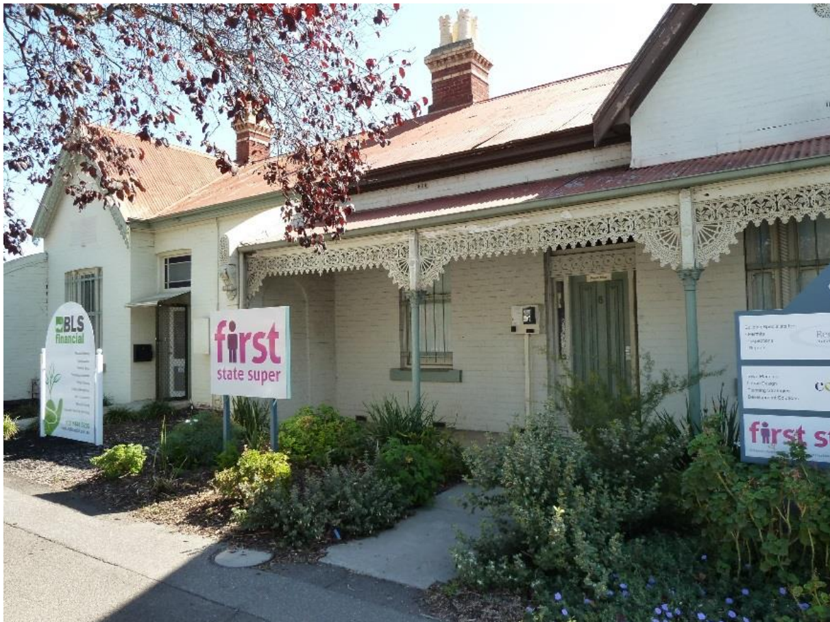
Figure 5 8–10 Garsed Street, Bendigo, as of 2016. (Source: Context, April 2016)
