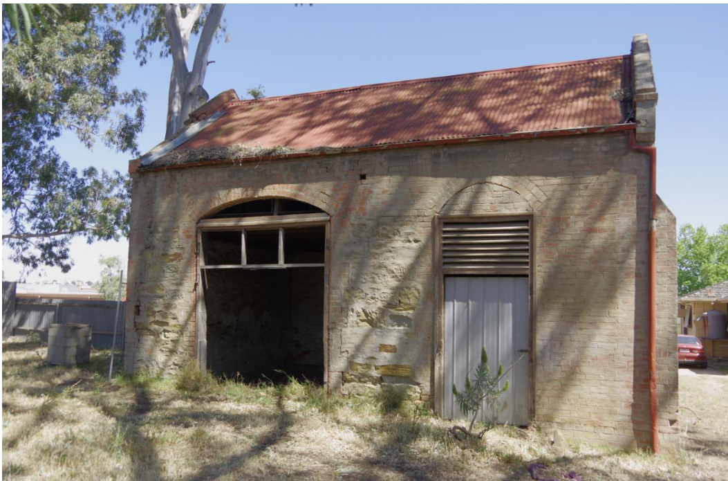
Figure 7. East elevation. Note: butresses to northern end of building and rubble stonework either side of wider opening. (Source: Context, November 2019)
