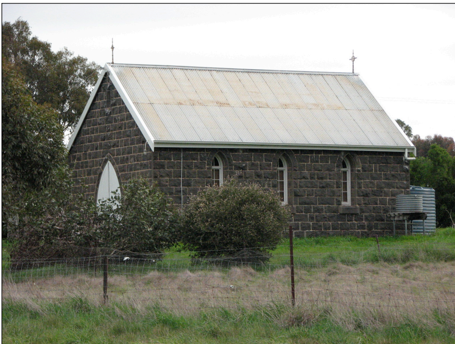
Figure 22: Church at Rossbridge, 2012. Photo by Tom Henty.
