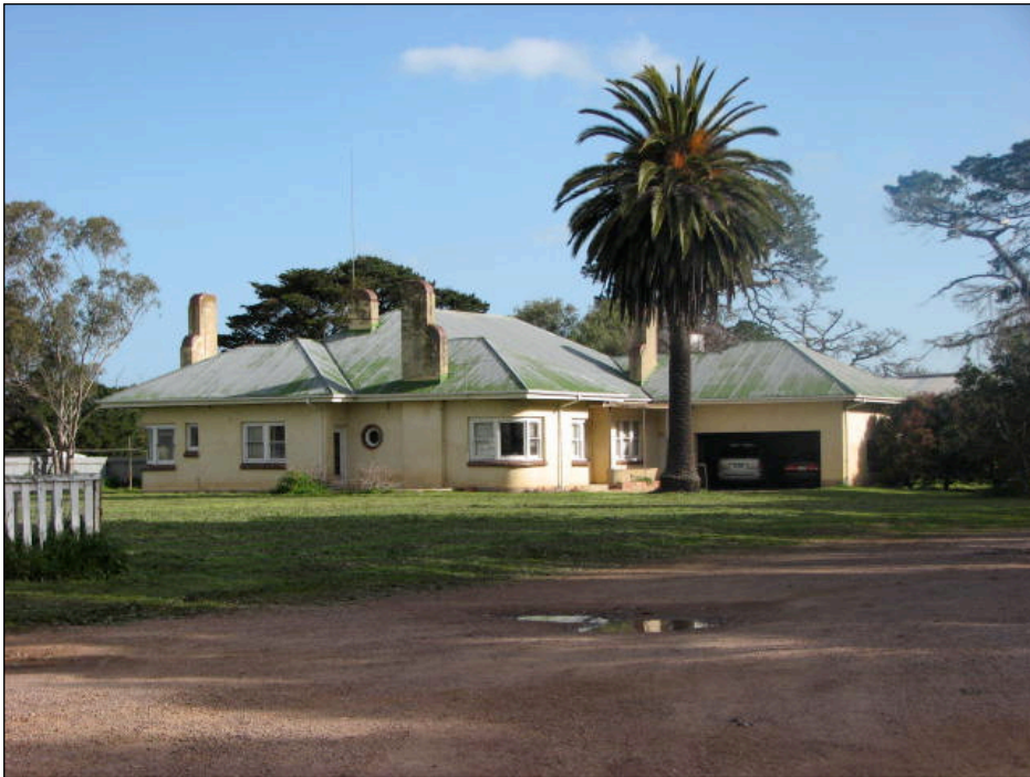
Figure 8: Residence built ca. 1953, Willaura, 2012. Photo by Tom Henty.
