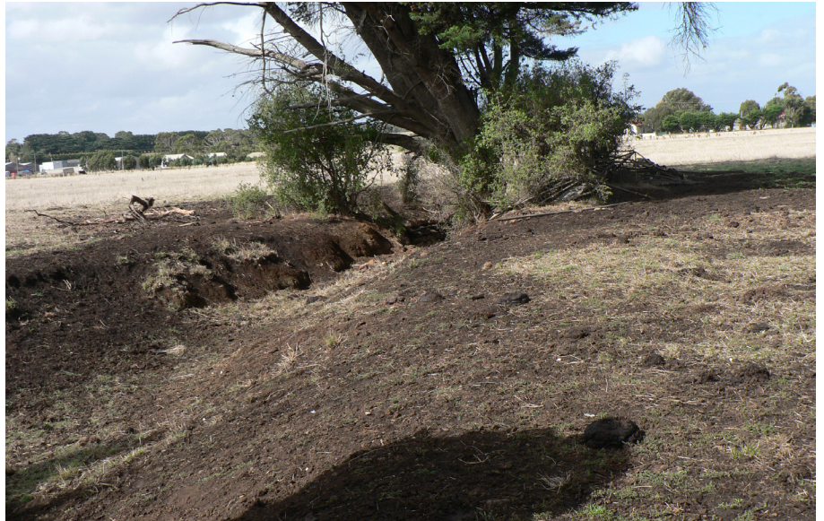
Unformed overland drainage line
