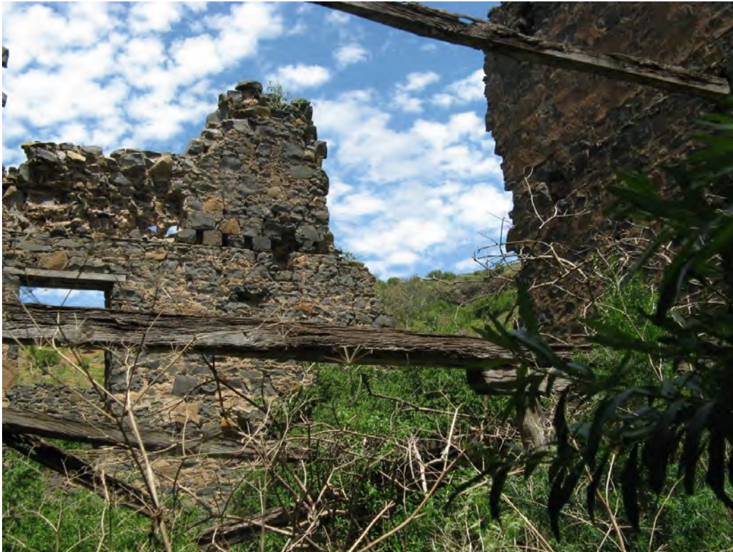
Photo 23: Interior of Lochton Mill, facing south (W. Anderson, 16/11/11)
