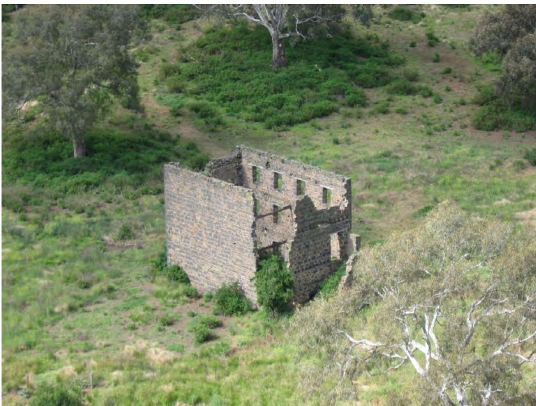
Photo 20: Lochton Mill viewed from the south, facing northeast (W. Anderson, 23/11/11)
