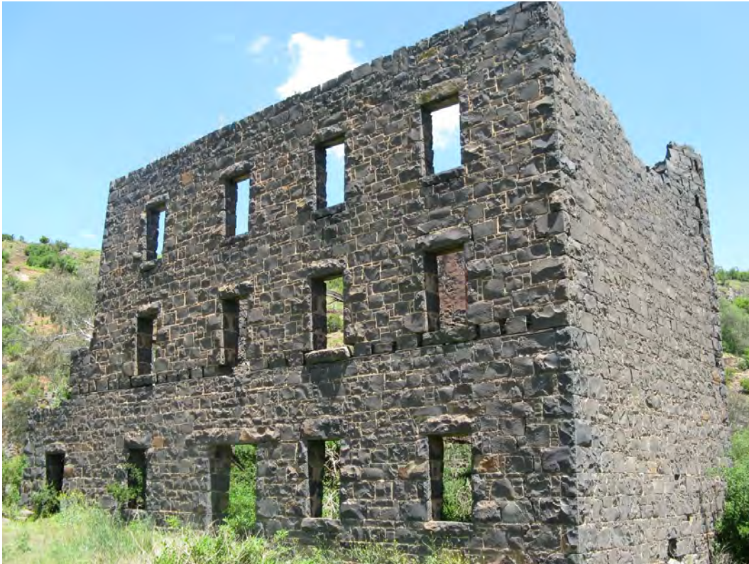
Photo 21: East front of Lochton Mill, facing southwest (W. Anderson, 16/11/11)
