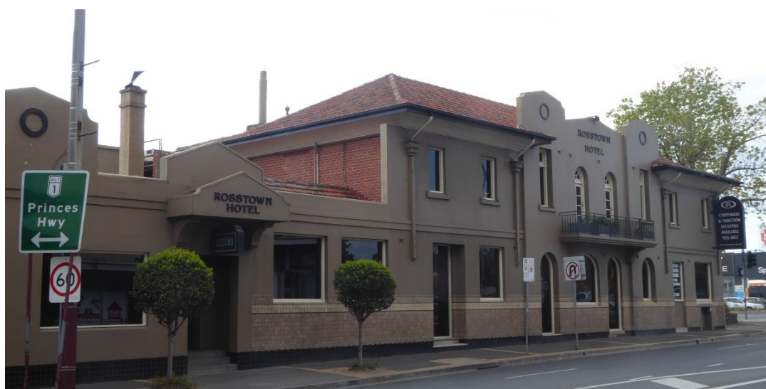
Koornang Road façade, 2018. The extent of the original part of the building can be seen by the dado tiling, the terracotta roofs, and the chimney to the original lounge. Note the horizontal parapet to the single storey section. RBA, 2018
