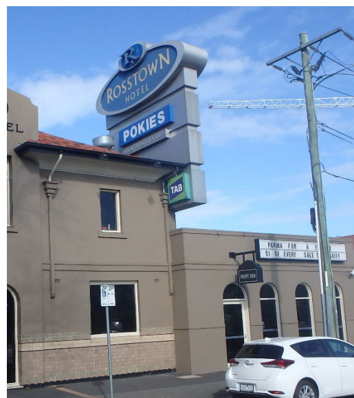
Recent signage to parapet of original building. Note that the eaves and downpipe abut the parapet/signage, and do not return around the corner. (Source: RBA 2018)
