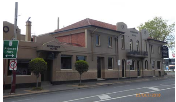
Figure 9: Rosstown Hotel viewed from Koornang Road.
