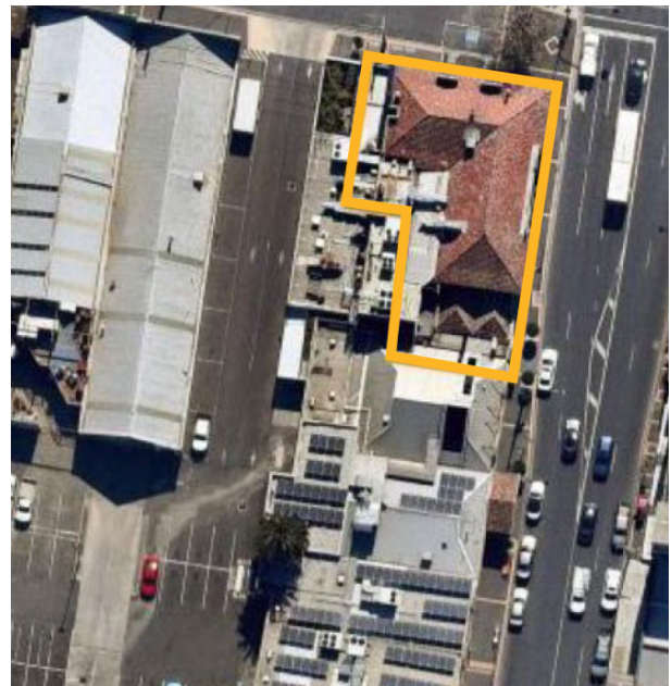
Figure 8: The significant heritage building on the Rosstown Hotel site is the building covered by the terracotta roof (both double and single storey sections). A 5 metre wide buffer (yellow line) to the south and west of the terracotta roof completes the mapped extent of the Heritage Overlay.
