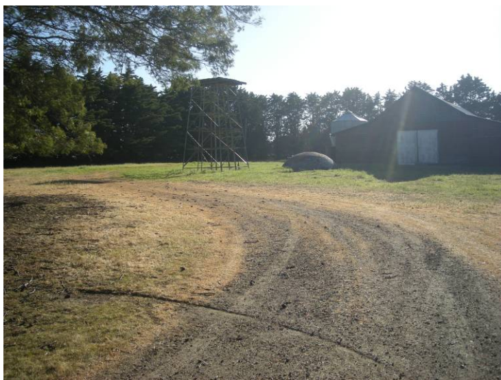
Plate 5 N6 Walton's Road Complex, showing a shed, water tower platform and corrugated iron shed
