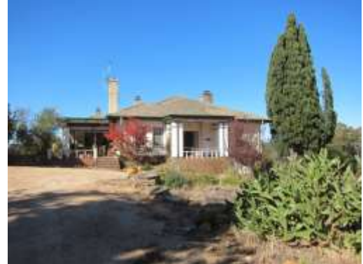
125-133 McIvor Road, East Bendigo, porch and main entry
