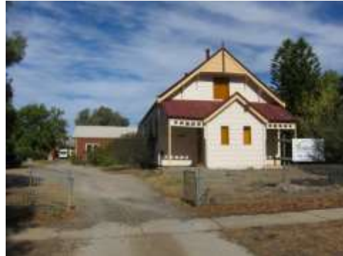
Church hall 60 Raglan Street, White Hills
