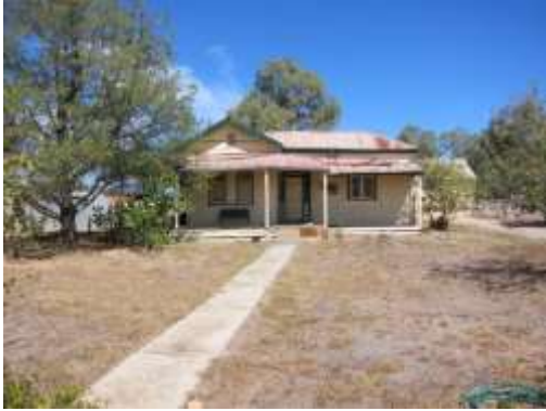
14 Heinz Street, White Hills, house
