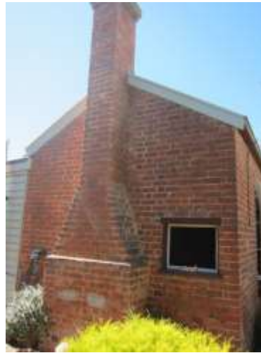
Kitchen and chimney at rear of house
