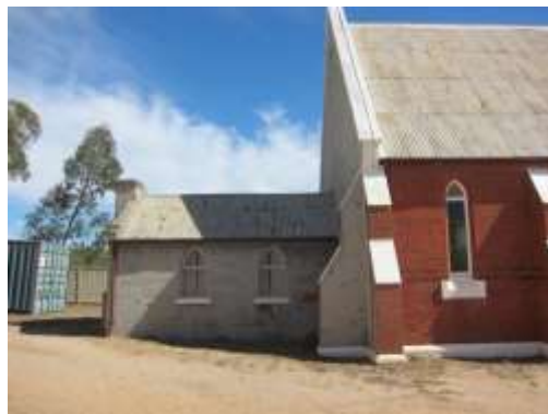
Vestry and possibly early Methodist Church c 1864 behind the later church
