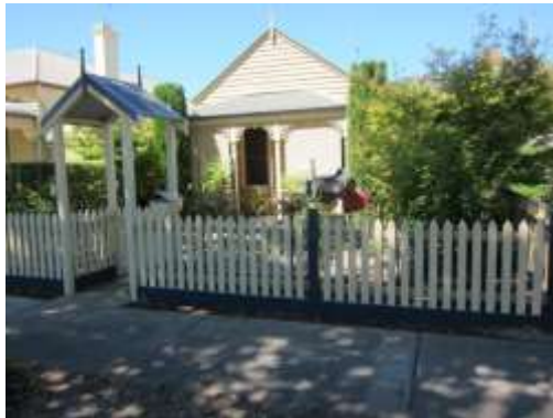
80 Bridge Street, Bendigo
