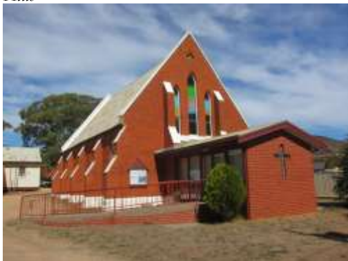
Uniting , former Methodist Church with contemporary porch built in front.
