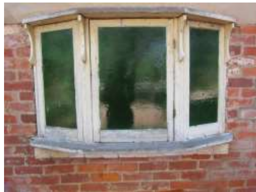
Detail of window added c.1920
