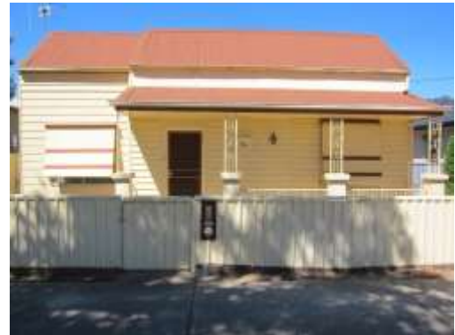
86 Bridge Street, Bendigo
