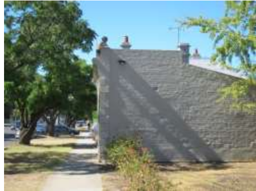
105 Lucan Street, North Bendigo, view from western boundary
