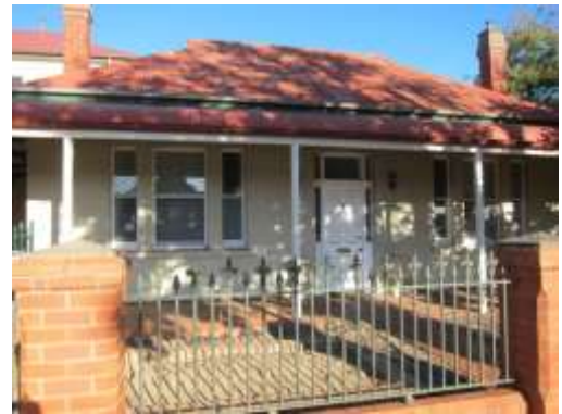
4 Weeroona Avenue, North Bendigo, house at front of site
